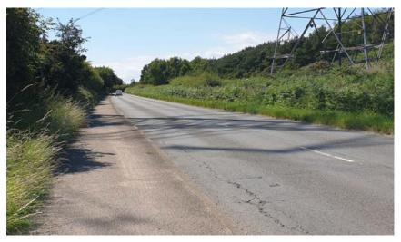
Looking west along Sizewell Gap road, an example of existing carriageway failure
